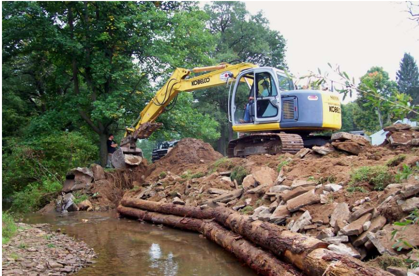
Above—Installation of modified mud-sill on Blacksmith Run
