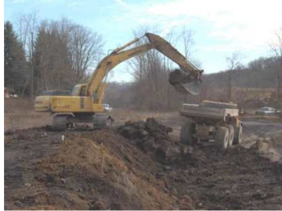
Construction of JB#1 Site Underway
