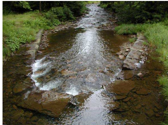
Engineered Rock Cross Vane, Big Bear Creek, Lycoming County
