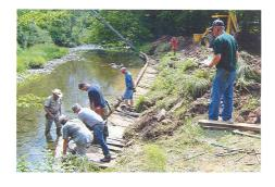
Additionally, a 130 foot mud sill with a 30 foot wing logs and multi-log vane deflectors was installed on kettle Creek in Clinto County near the village of Cross Fork as a separate project sponsored by the <u>Kettle Creek Watershed Association</u> and the Kettle Creek TU Chapter.
