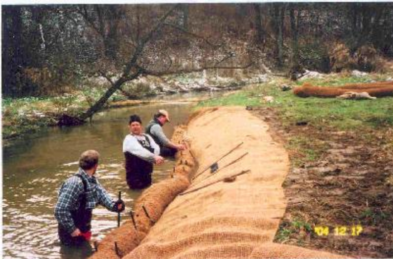
Fiber matting and bio-logs to stabilize stream bank.
