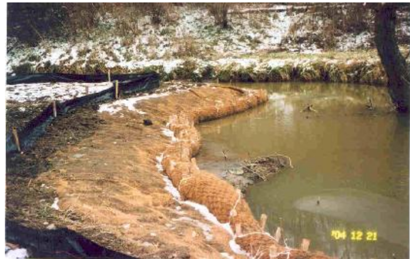
Stream bank is now ready for Spring planting.
