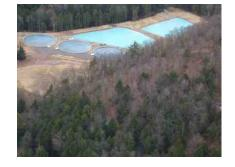
This system passively treats up to 14,000 gallons per minute of acidic mine water discharging from the Audenreid Tunnel. In terms of amount of water treated it is the largest passive AMD treatment system ever built in Pennsylvania and perhaps anywhere.
