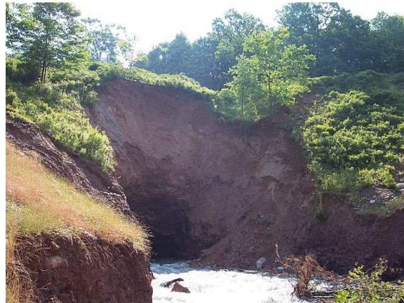
Flooding Blew Out the Audenreid Mine Discharge Tunnel Where It Attached to the Newly Dedicated Treatment System in Schuylkill County.
